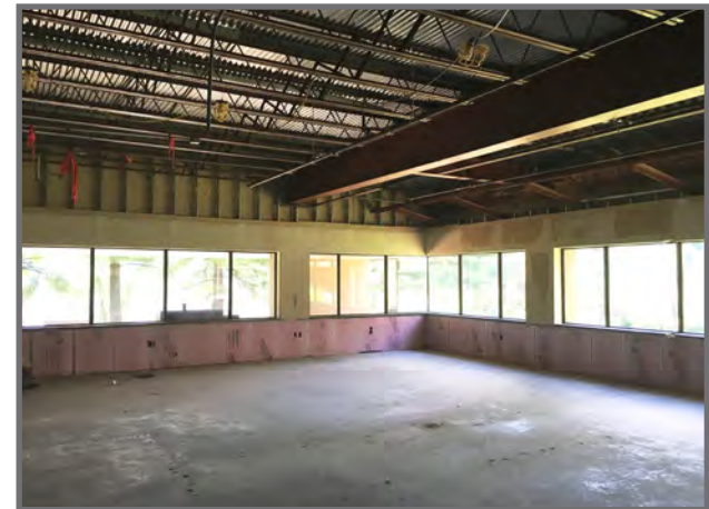
Exposed Ceilings - Corner Suite
