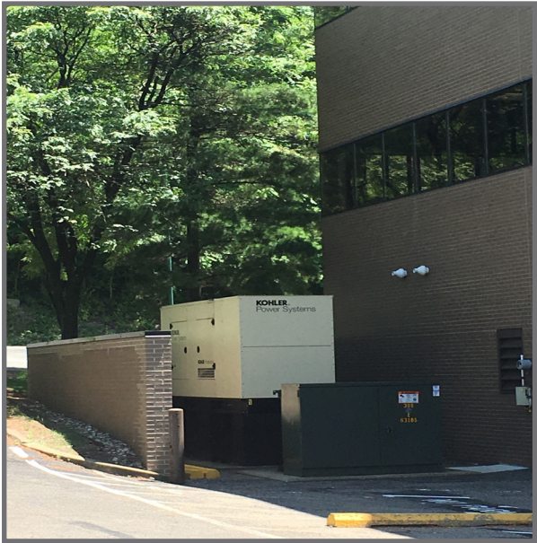
Back-Up Generator (200 KW, 301 AMP Diesel)
