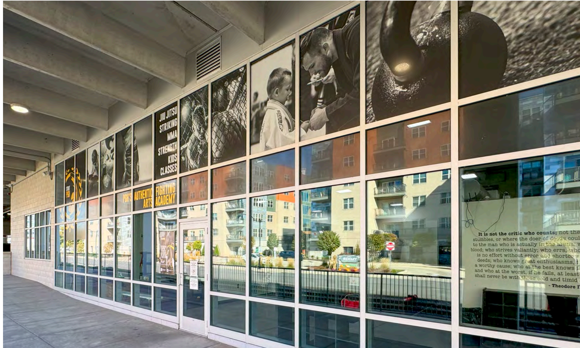
Walkway and Entrance Facing West
