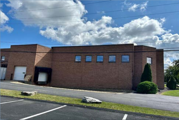
Grade Level & Dock Access
